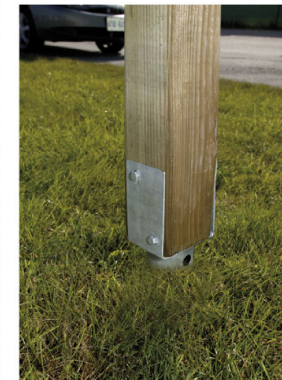
Step 2 Secure 4x4 wood post with lag bolts.
